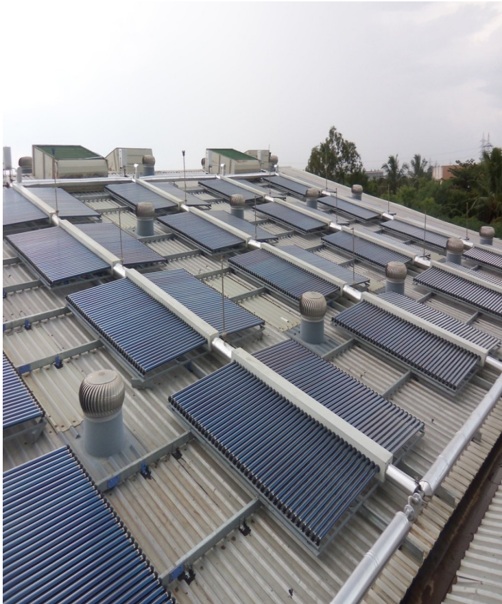
210 KW Solar Thermal System – SONA KOYO STEERING SYSTEMS LIMITED
