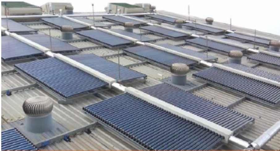
Solar Thermal System Installed on trussed factory roof top.
